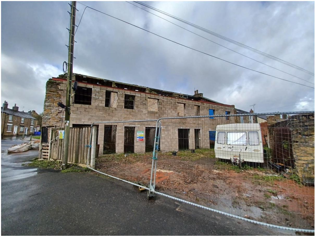
Photo 2: Rear elevation of application building.
