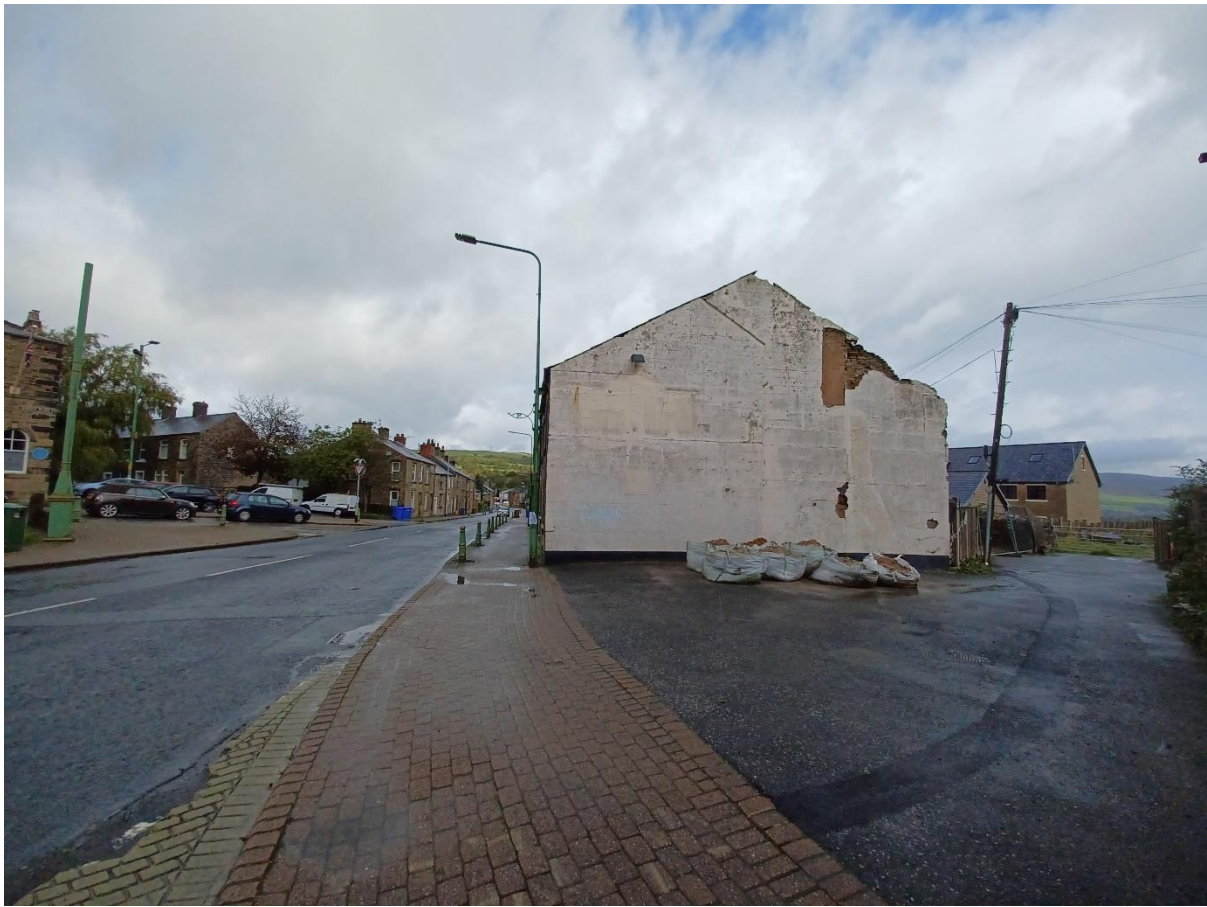
Photo 3: Side elevation of application building.
